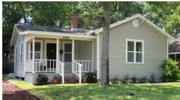
Murray Hill House After
